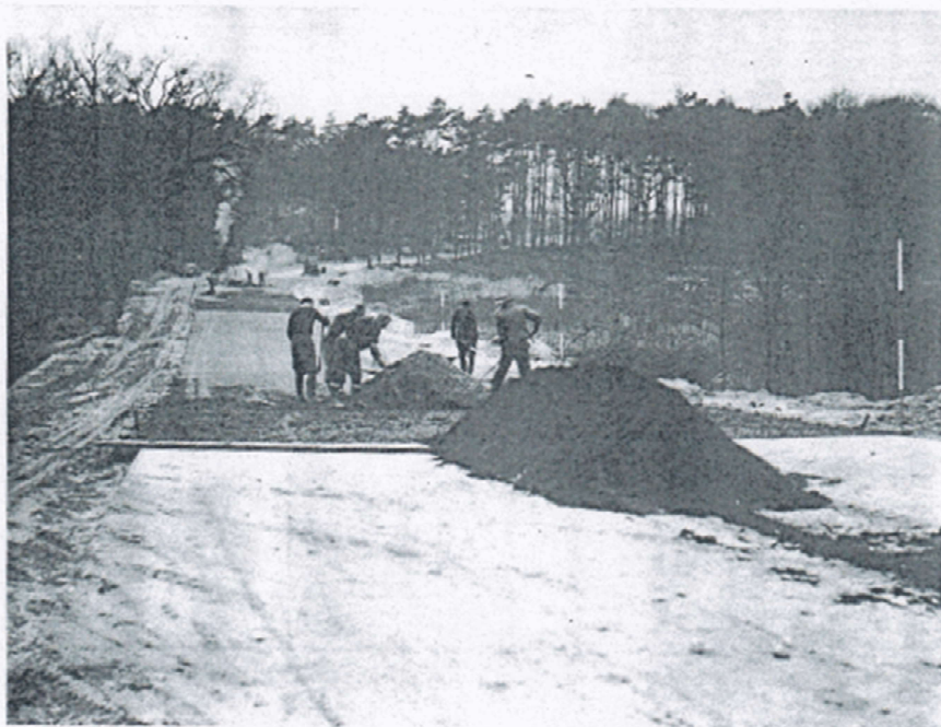
Photo 14.—Laying the first roads.
